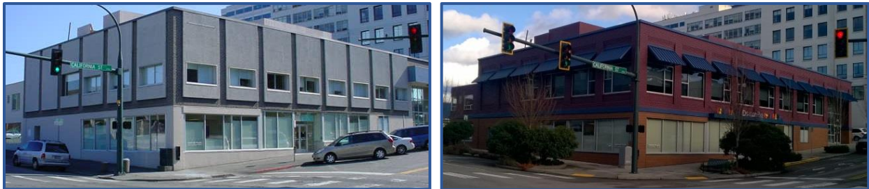
Dawson Place Child Advocacy Center: before (left) and after (right) renovations
